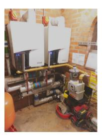
It is recommended that these areas of expose pipework and fittings are insulated with bespoke made flexible insulation jackets. These wrap around
